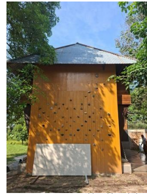
Gambar 8. Arena Wall Climbing Sesudah
