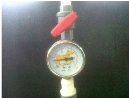
GAMBAR 3. PENGECEKAN BALL VALVE
