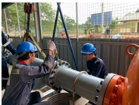
Gambar 1. Kegiatan Cleaning Metering System
