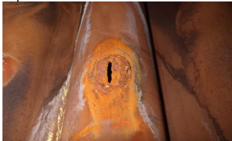
Gambar 6. Pipa Boiler Pecah
