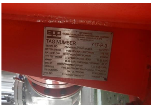
Gambar 2. Data sheet Fire Pump 717-P-3
