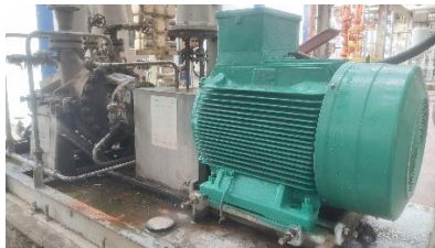
Gambar 5. HP Carbamate Pump (D2-307-J-K2)
